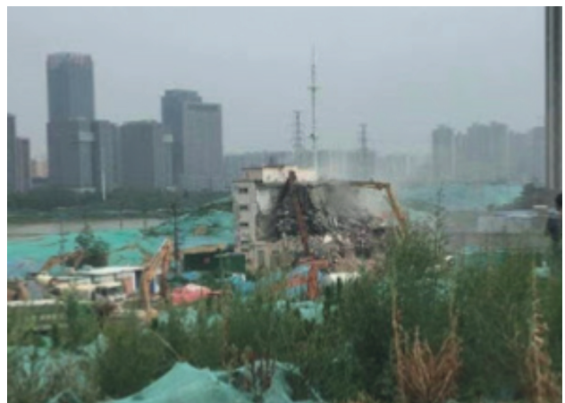
CCP destroyed Sunzhuang Church; injured Christians (hospitalized).
