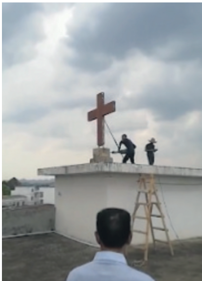
CCP authorities contracted men to remove the cross from Xiaohe Christian Church.
