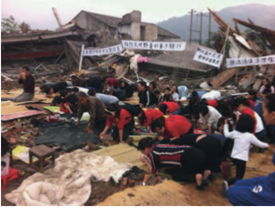
Example of increasingly commonplace church demolitions.
